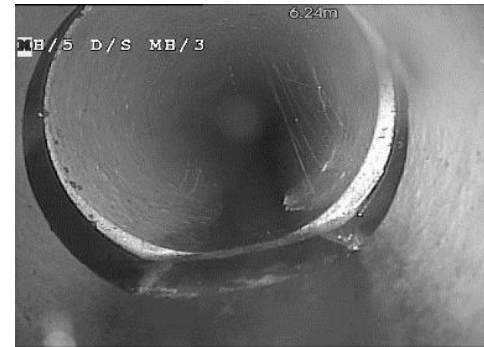
Displaced Joints
