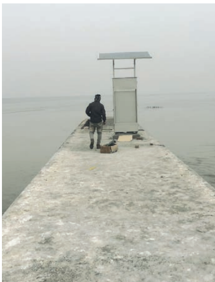
s::can Monitoring Station
